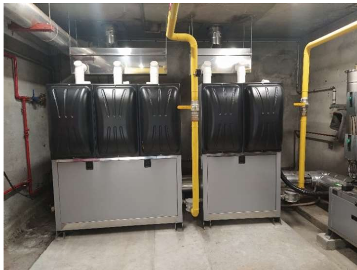
Fig.7 – Modules chaudières TERRIS ENERGIE T-EASY 5x125kW
