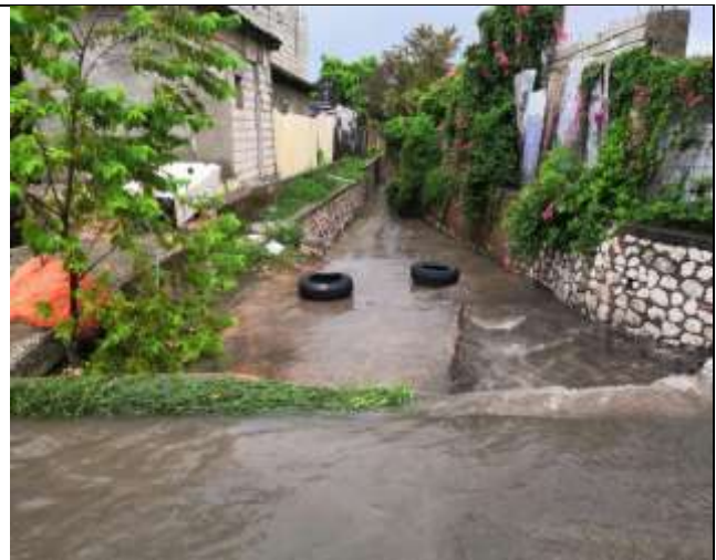
Figure 4.20: Photo of runoff sheet flowing from the road to the gully servicing the Clifton cathcment area.
