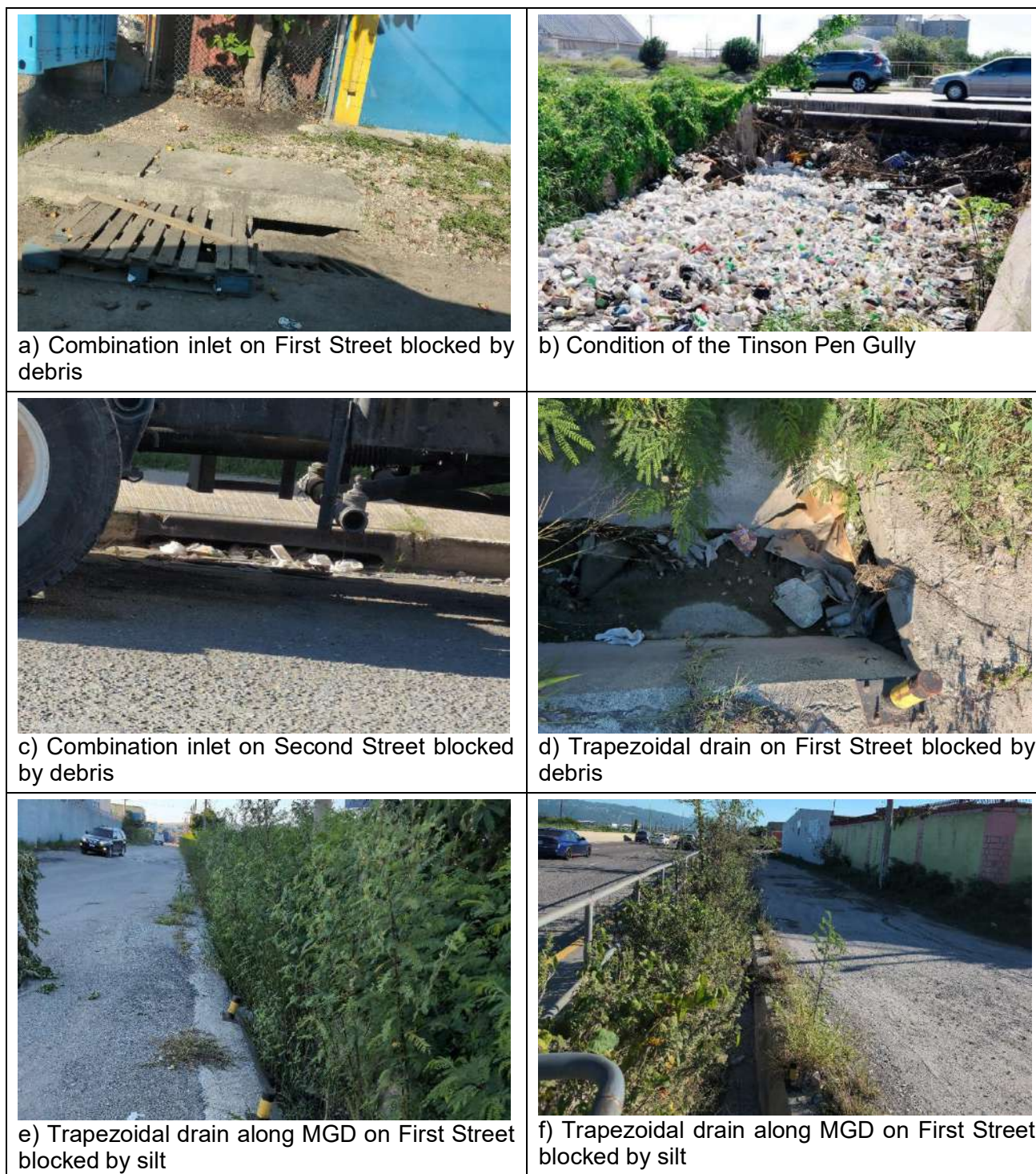
Figure 14: Condition of the existing drainage in the Newport West and Marcus Garvey drive area.
