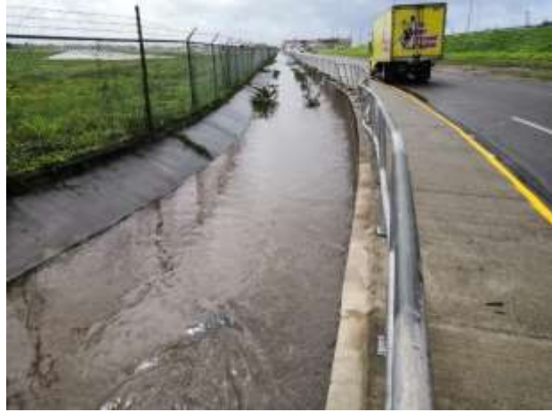
Figure 9.13: Marcus Garvey Drive drain during 1-2yr RP rainfall event
