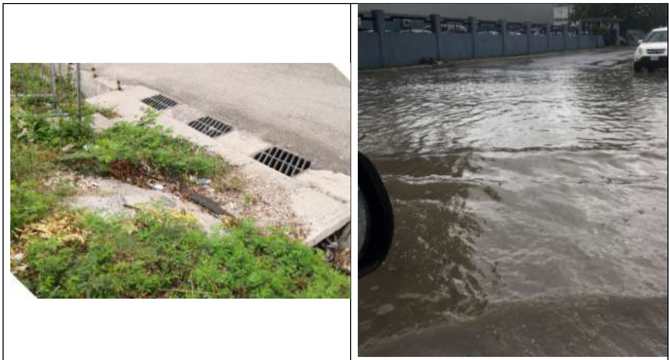
Figure 4.12: Photos of Newport West inlet during normal conditions, and during heavy rainfall (same location)
