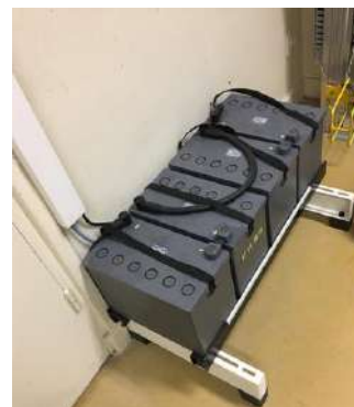
4x batteries 12 Vdc
