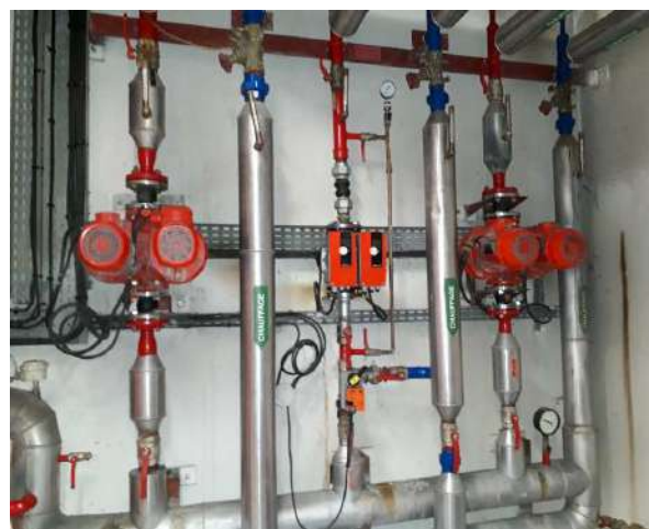
Panoplie hydraulique chauffage
