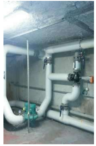
Panoplies hydrauliques chauffage
