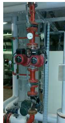
Panoplie hydraulique chauffage
