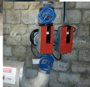
Panoplie hydraulique
