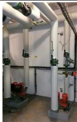
Chaufferie - Panoplie hydraulique
