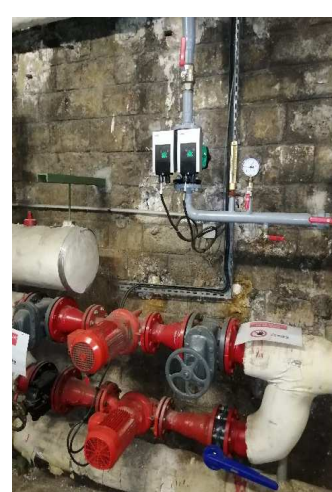
Panoplie hydraulique
