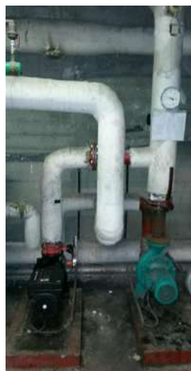
Panoplie hydraulique chauffage
