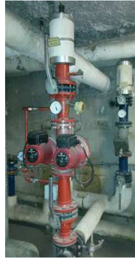
Panoplies hydrauliques chauffage
