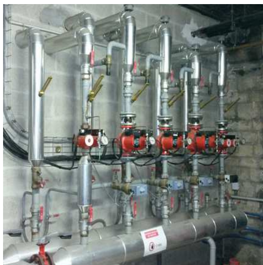
Panoplie hydraulique
