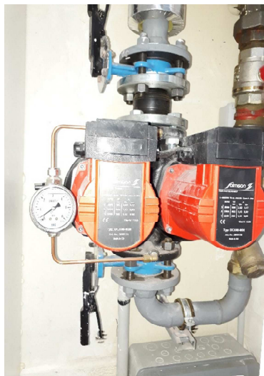
Pompes chauffage
