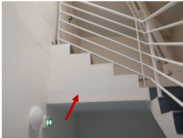
Fissure jonction dalle / chape
