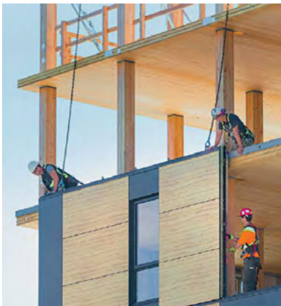
Structure mixte poteaux-dalles-FOB - Brock Commons Tallwood - AO Architects, Vancouver (ca)
