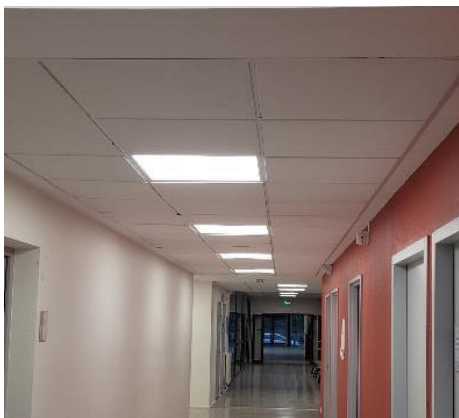
REPERE LUM 01 - Luminaire 600x600 - Circulation
