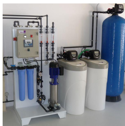
FIGURE 4 - EXAMPLE OF OSMOSIS WATER TREATMENT
