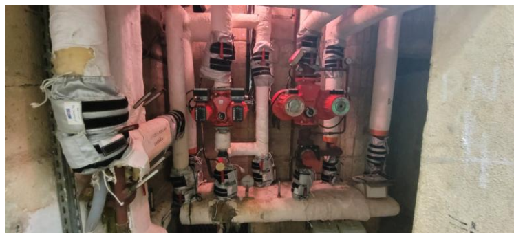
Figure 14 : pompes de distribution
