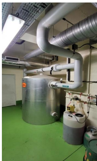
Figure 31 : ballon tampon
