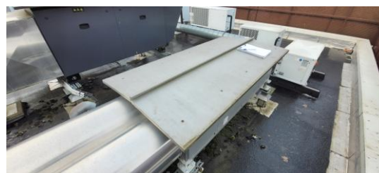
Figure 28 : CTA double flux
