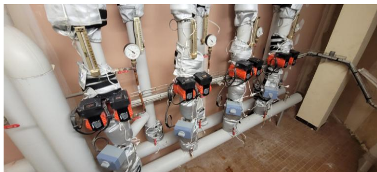
Figure 15 : pompes de distribution
