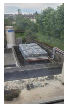
Figure 28 : Dry-cooler
