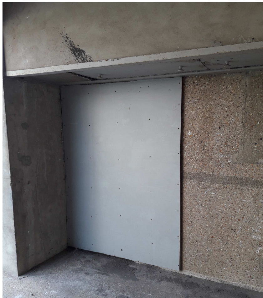
Façades (Enveloppe) - Plaque fibre ciment
